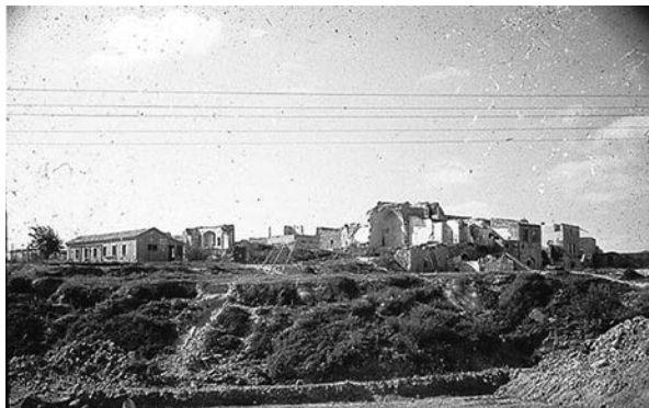
Figure 5.3. Start of excavations in Area A. Kaplan Archive.
